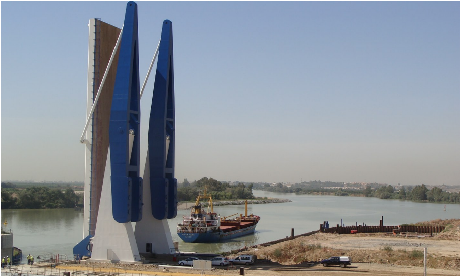
Seville harbour lock
