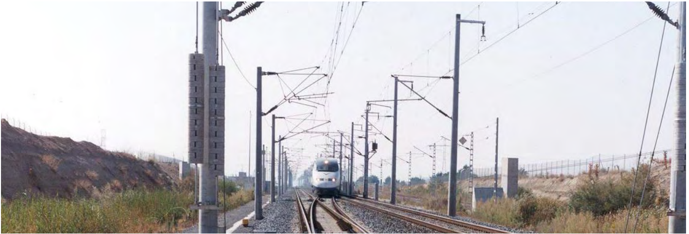
AVE high-speed railway line
